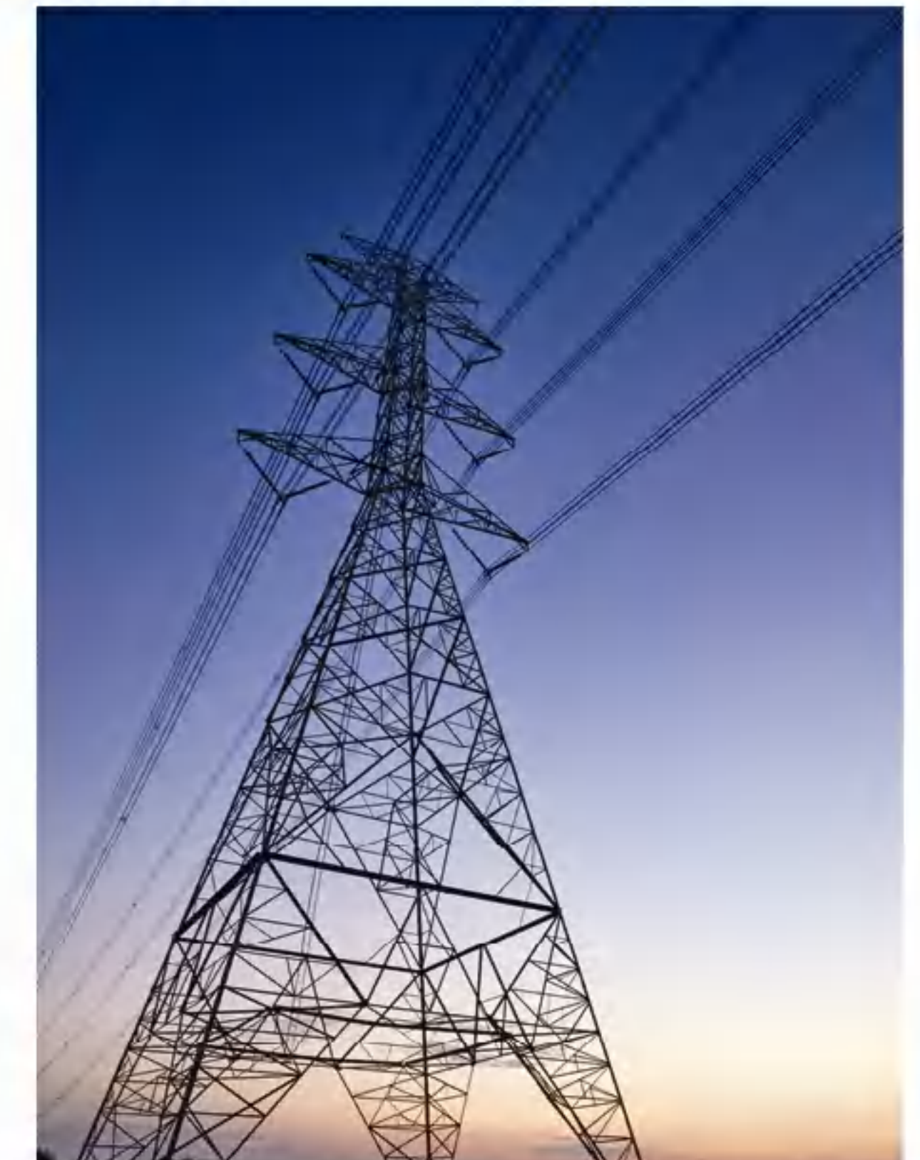
钢结构 Steel Structural Construction
