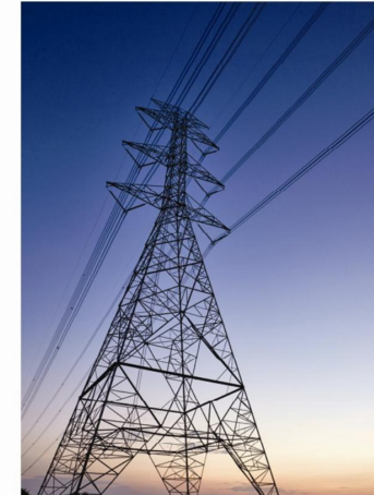
钢结构 Steel Structural Construction
